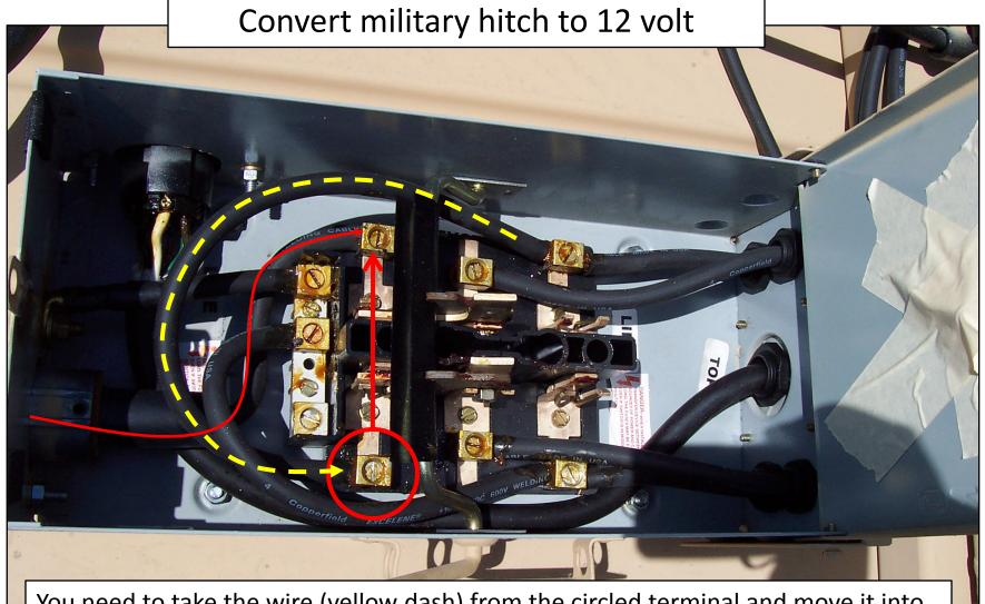
You need to take the wire (yellow dash) from the circled terminal and move it into the slot to join the feed from the receptacle. You will then set the box to 12volt and feed the cable from your truck into the box for 12 volt power. No longer use the 24 Volt handle position.
